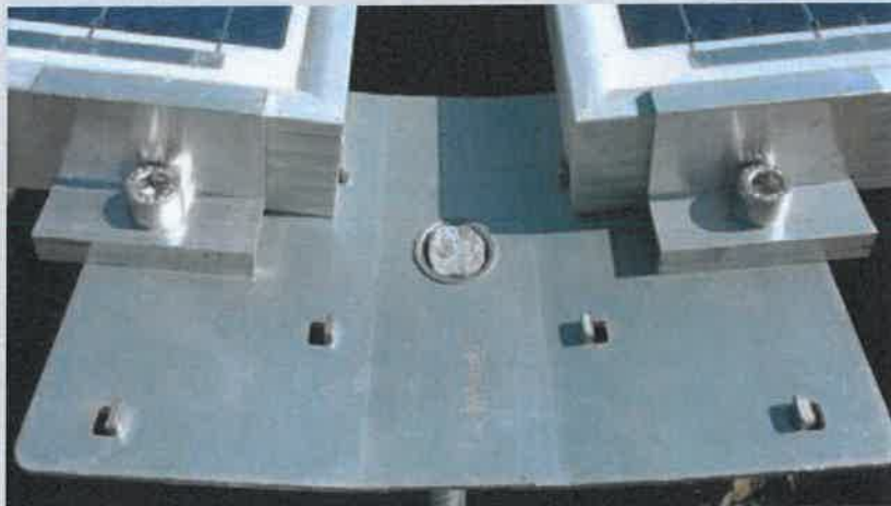
▶ Module mounting with Edge Clamp: At the North and South edges of the PEG block
