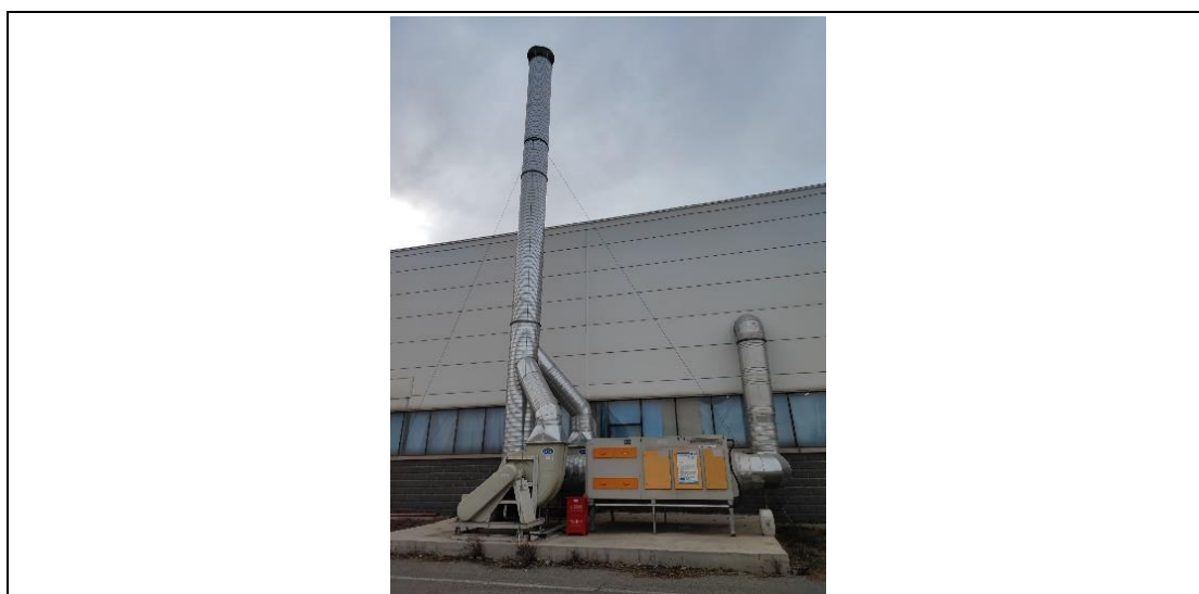
Photo-oxygen activated carbon integrated equipment adopted by the Tianjin Base to collect and treat workshop exhaust gas
