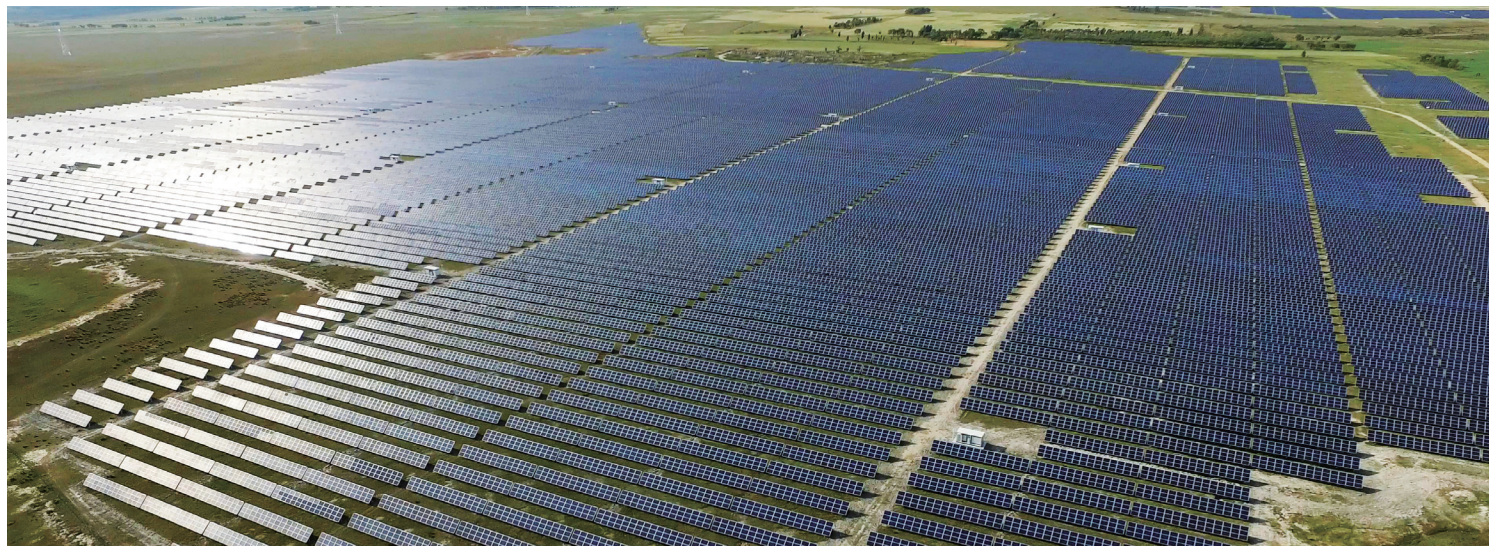
240 MW PV plant of Internet plus smart energy in Zhangbei County, Hebei Province, China
