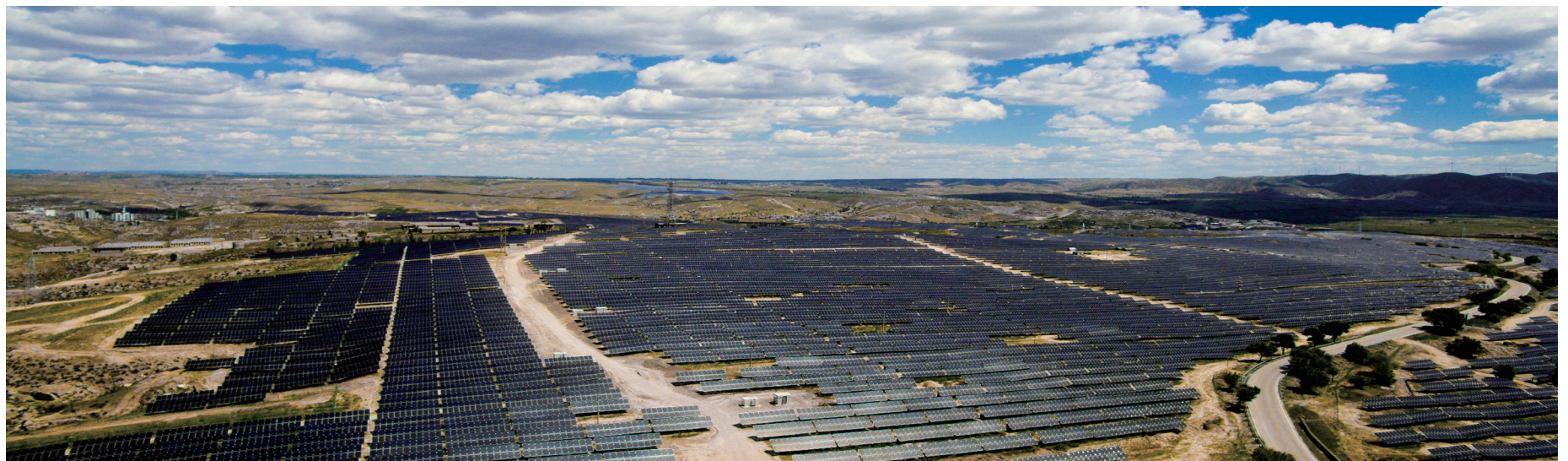
50 MW N-Type bifacial PV plant of national "Top Runner" advanced technology demonstration base in Datong, Shanxi Province, China
